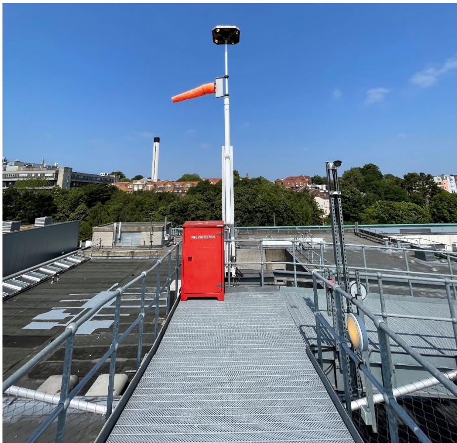
Figure 4-6: Photograph of windsock
