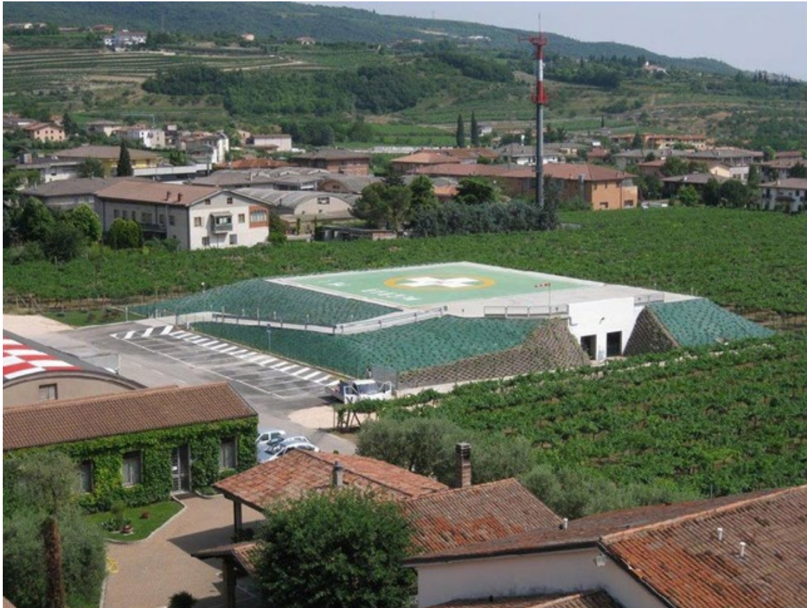
Figure 8-2: A mounded heliport at surface level (Ospedale Negrar)
