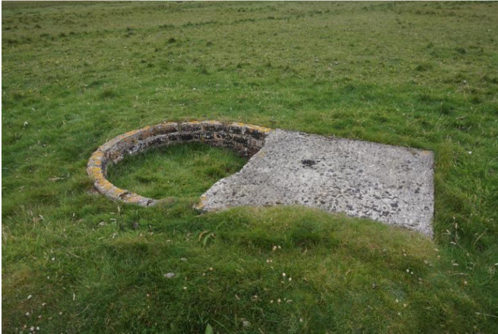
The concrete roof is partly covered with turf.
