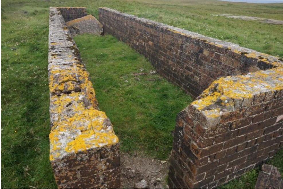
General internal view from south.
