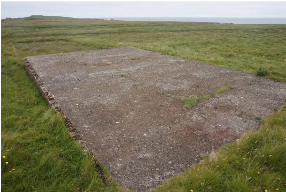
General view from northwest of west portion comprising concrete floor slab surrounded by part buried brick footings.
