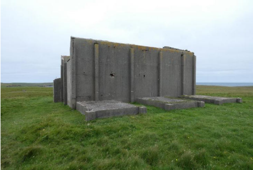
South elevation. See photos 2 and 4. This wall is a tall, thin, free-standing element.
