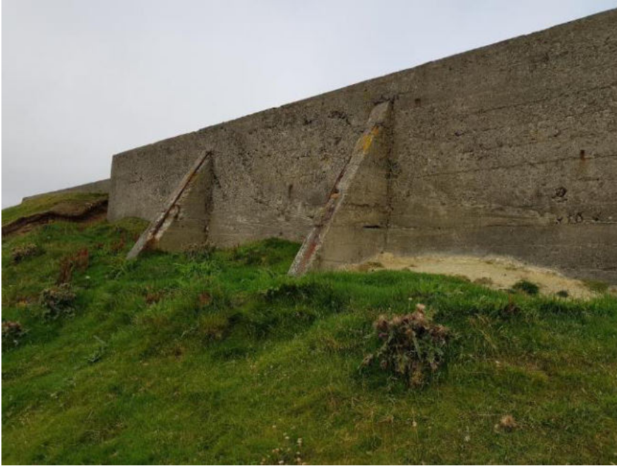
RC buttresses to the blast walls of the south side of the structure.
