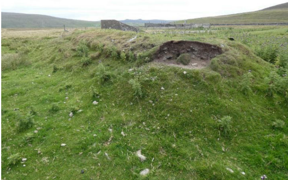
General view from southeast. Note damage caused by grazing and burrowing animals. Replacing the missing and damaged earth and turf banking will protect the structure below.
