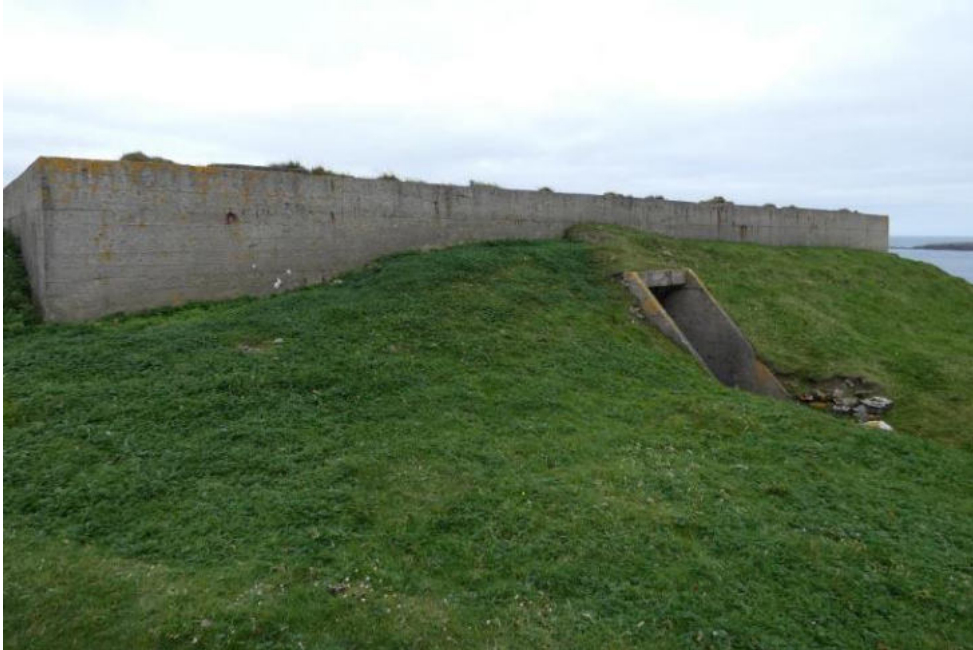
General view showing the embankment against the blast walls.
