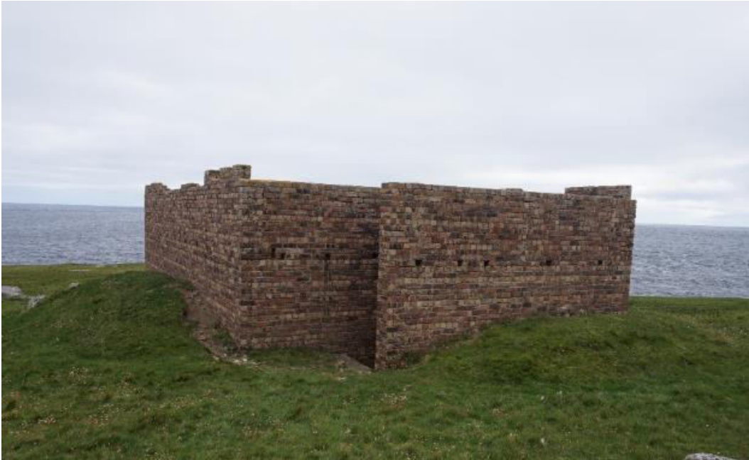
Fig.1: Blast walls were constructed in brick with sloping earth banks externally to protect temporary timber operational buildings of the Advance Home Chain.
