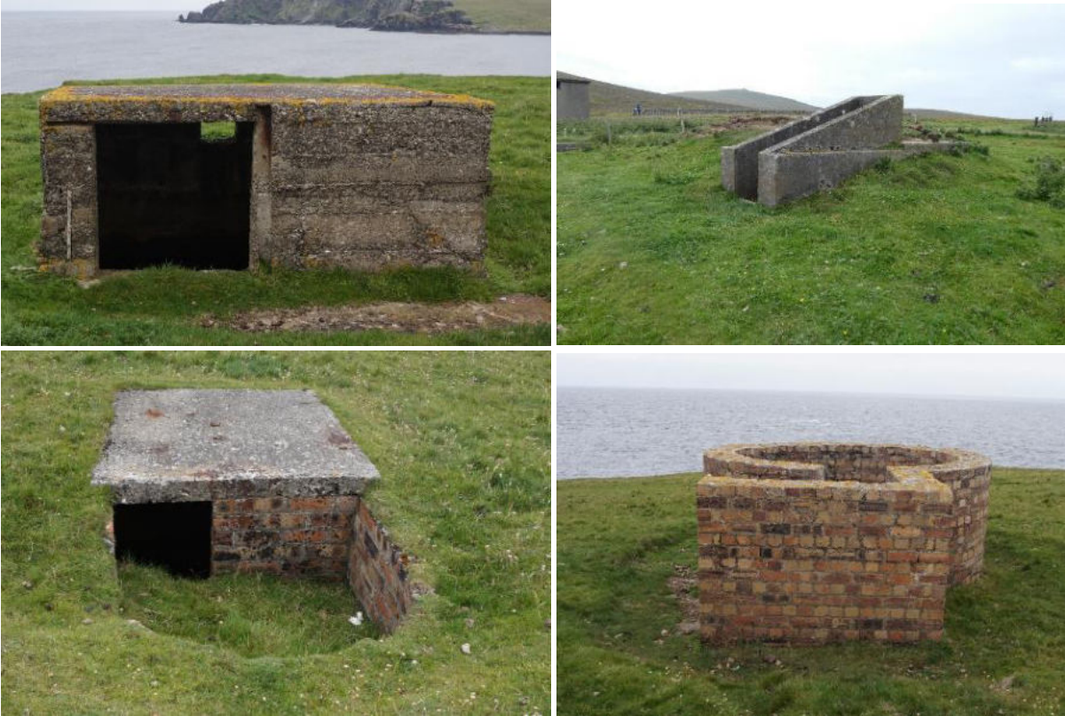
Figs. 3 to 6: Defensive structures comprise brick and reinforced concrete, most with additional earth and turf protection.
