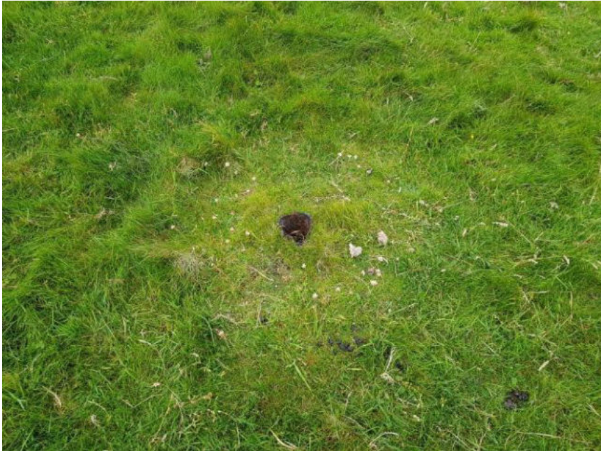
Projecting remains of a former camouflaging netting support post. The posts are severely corroded with sharp jagged ends.
