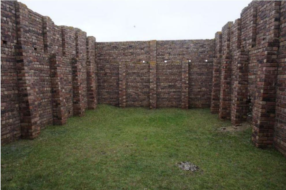
Internal general view.
