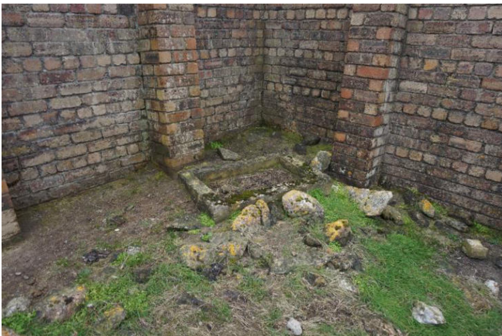
The small rectangle brick structure internally is in good condition. There are loose stones and bricks throughout the grass covered floor internally.
