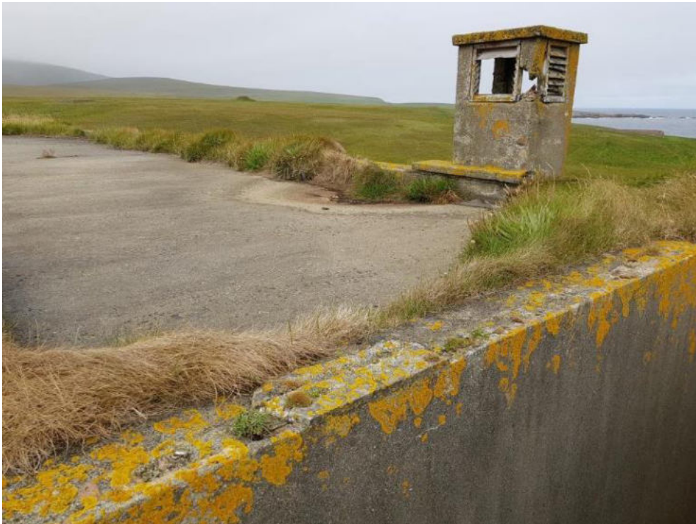
As 6. Note broken leg of RC cap to chimney – see next photo.
