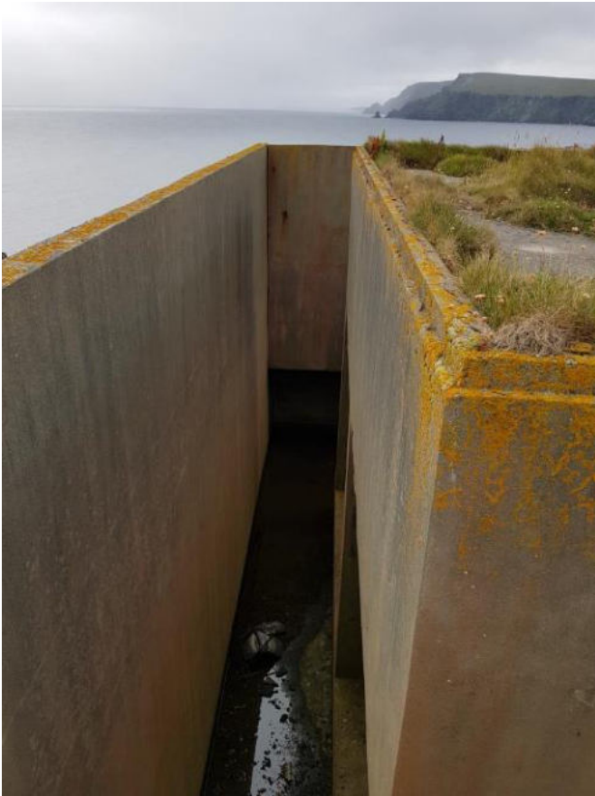
From the top of the embankment looking down into the lightwell between the blast walls and building proper.
