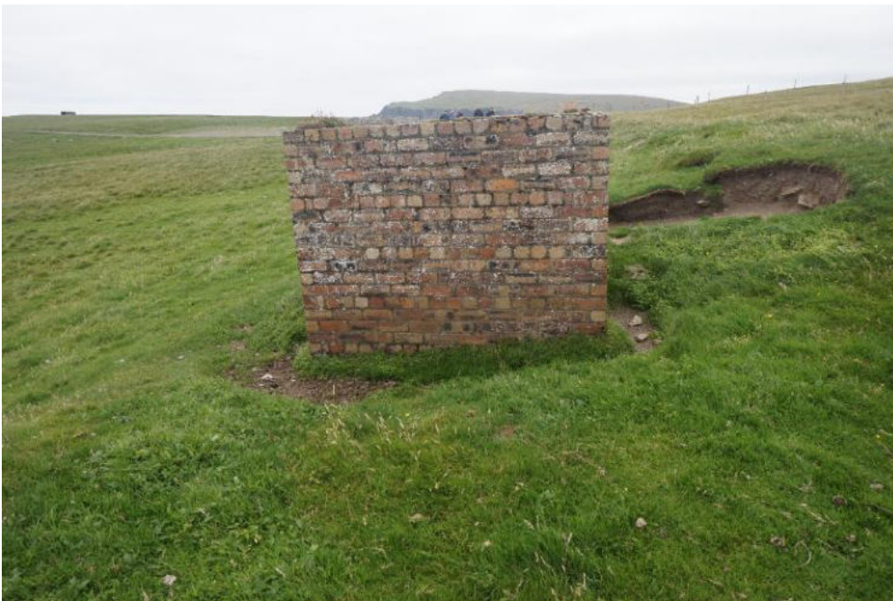
No structural cracking was observed despite the walls not being plumb or level.
