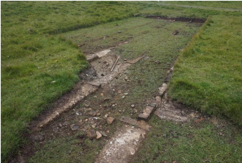
Loose brick footings, disaggregated concrete strip foundations and displaced bricks, timber and metal work at southern portion of the structure.
