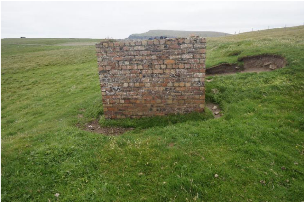
No structural cracking was observed despite the walls not being plumb or level.
