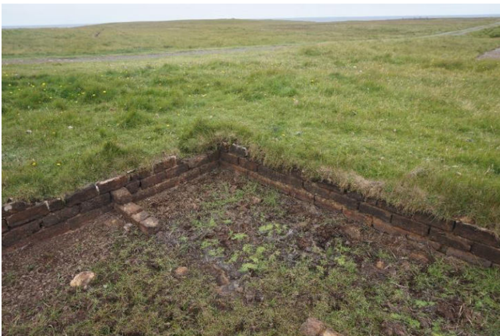
Part buried footings with loose bricks and failing mortar joints in northeast corner.
