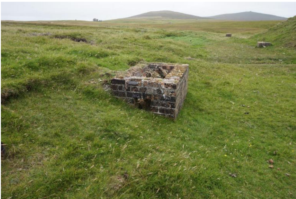
View from east showing small opening at ground level.
