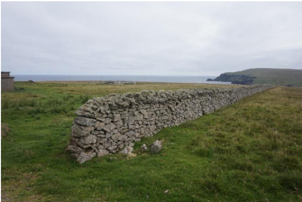
General view south: Copes should be regularly check and loose/displaced stones reset.
