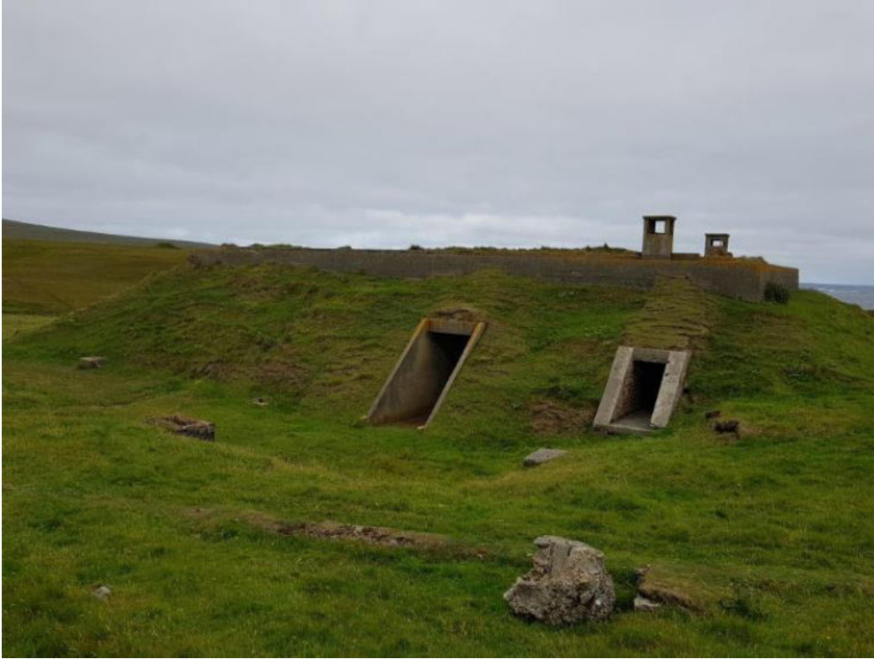
South side of the building. Note duct tunnel adjacent to entrance tunnel.
