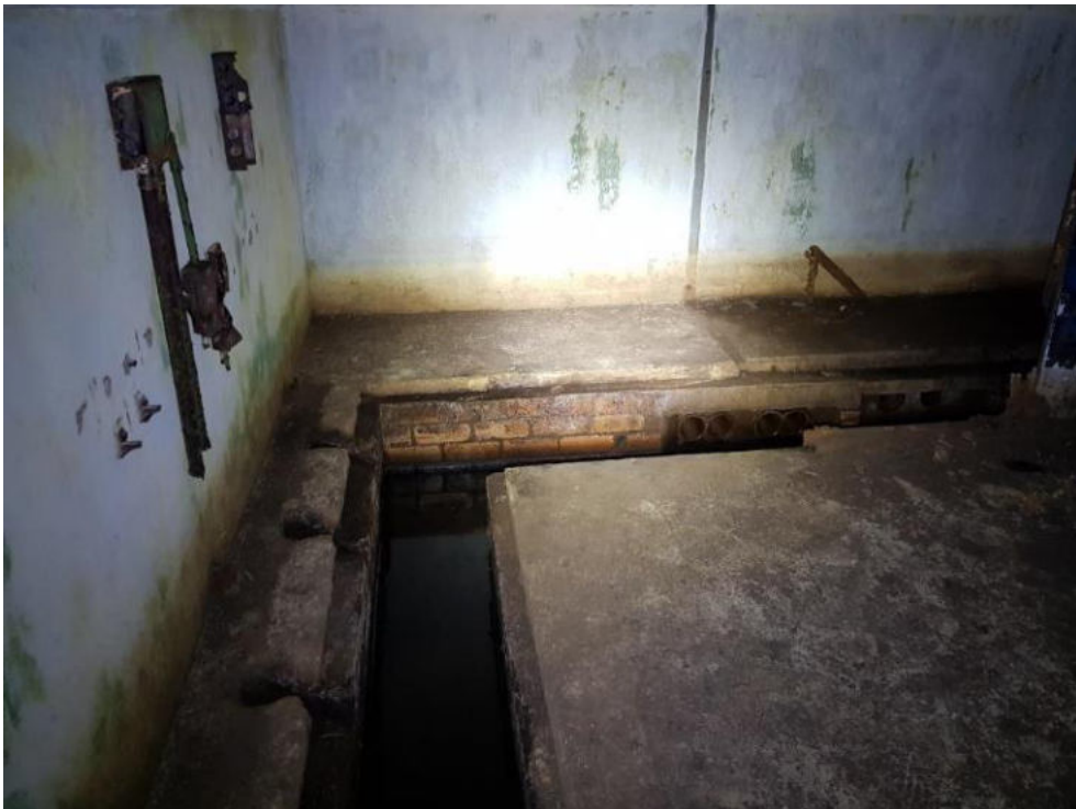
Open floor trench.
