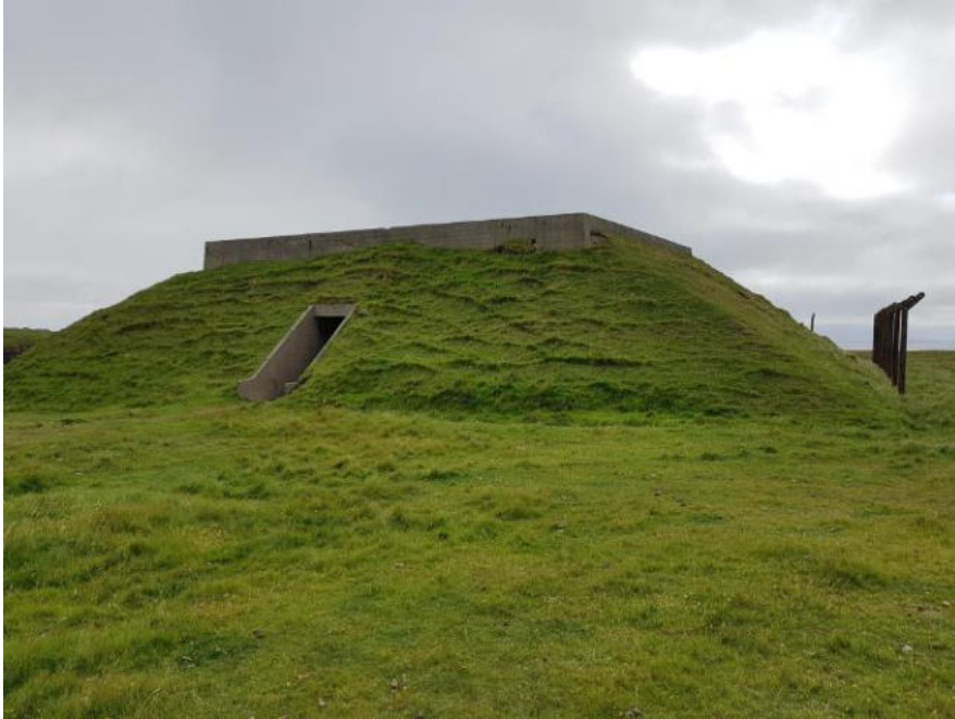
General view of the structure. The embankment is laid against RC blast walls about the building itself.
