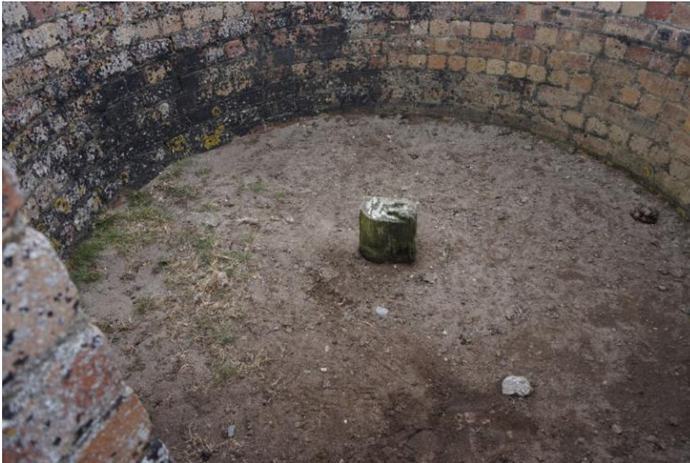
Partly obscured internal floor with central timber post.
