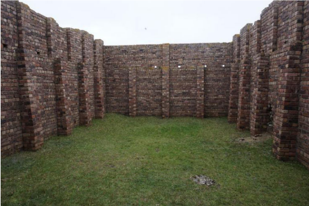
Internal general view.
