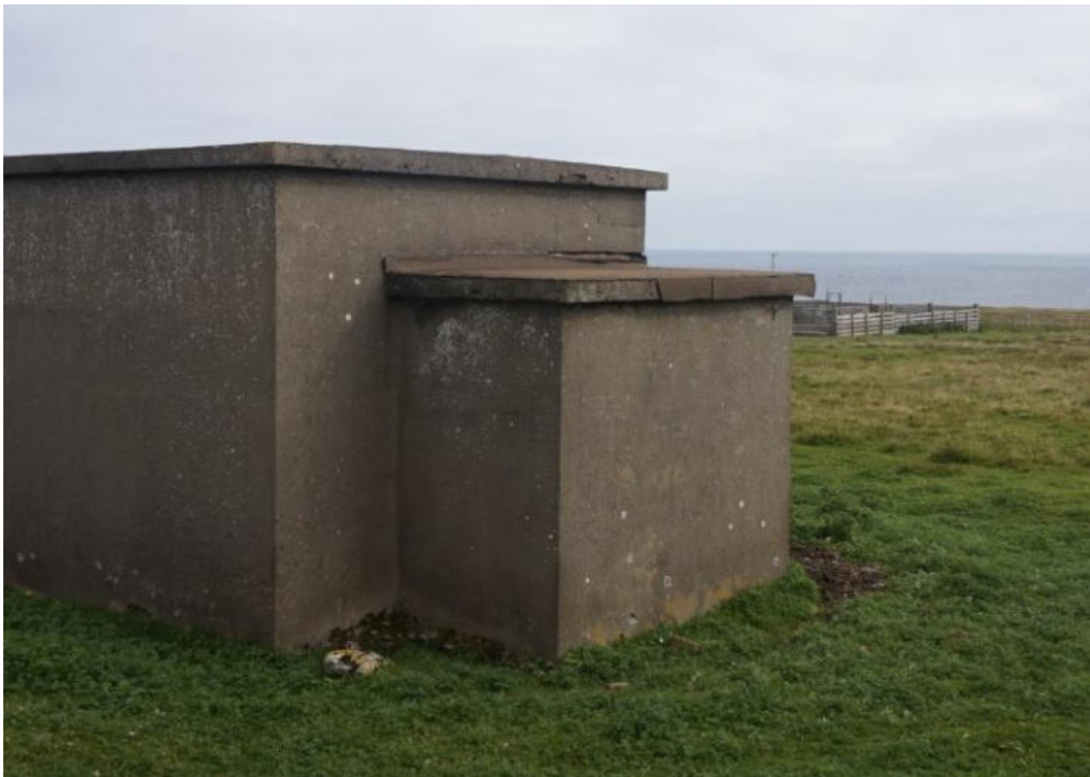
Failing asphalt junction between the west entrance porch and main building. Only fragments survive on the main roof.
