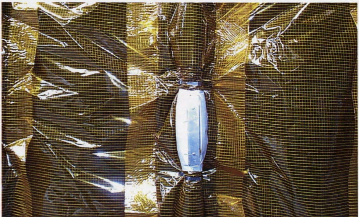
Figure 28 Simulated Clamp Block with Insulation Installed
