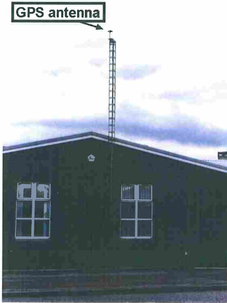
Figure 15 Onshore System Antenna
