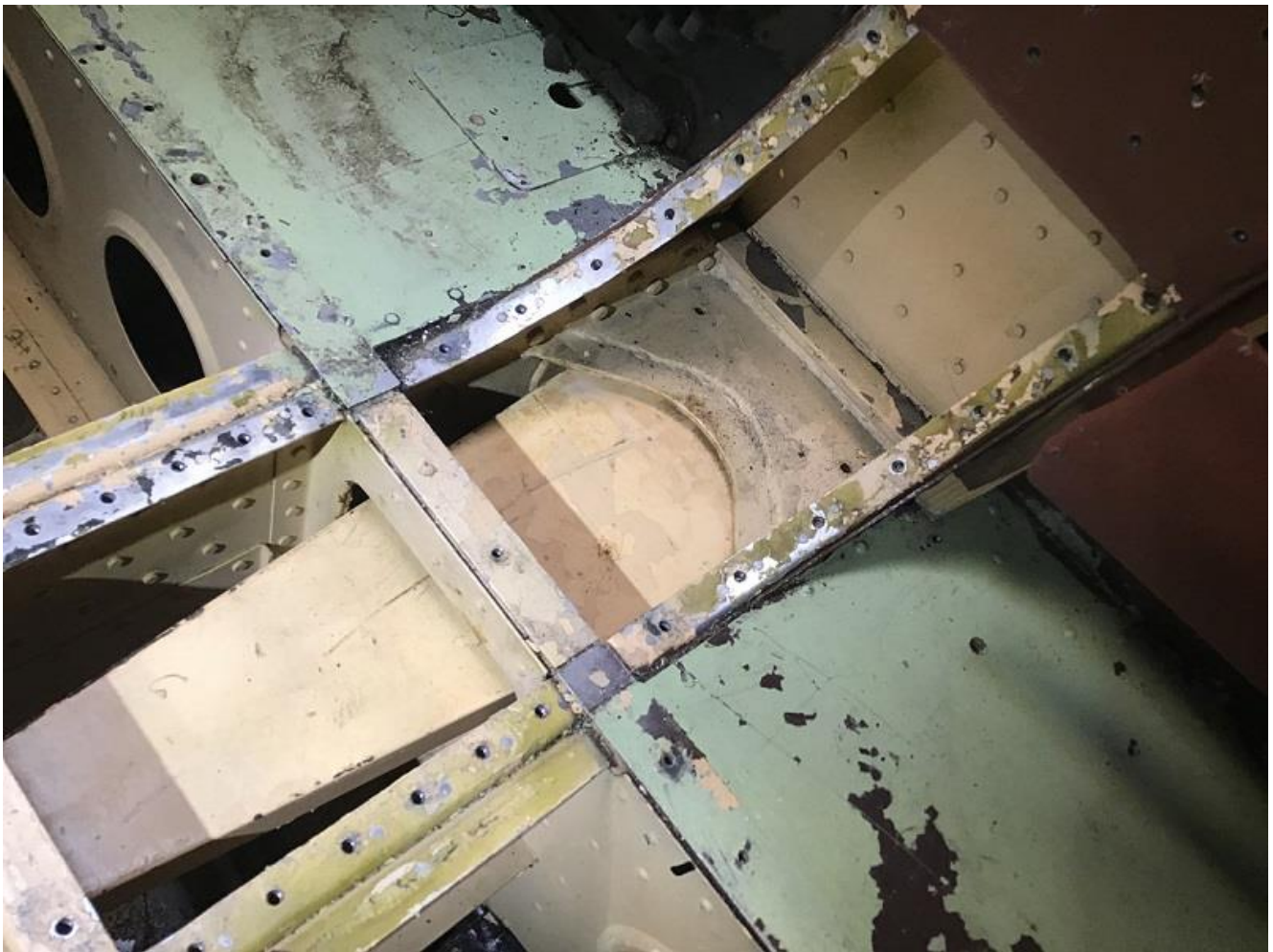
MH.1521 Starboard undercarriage support letterbox bracket. Undercarriage leg still fitted
