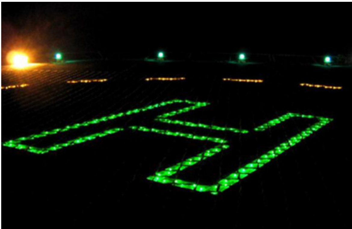
Figure 11 Heliport Identification Marking ('H') on the Thames A
