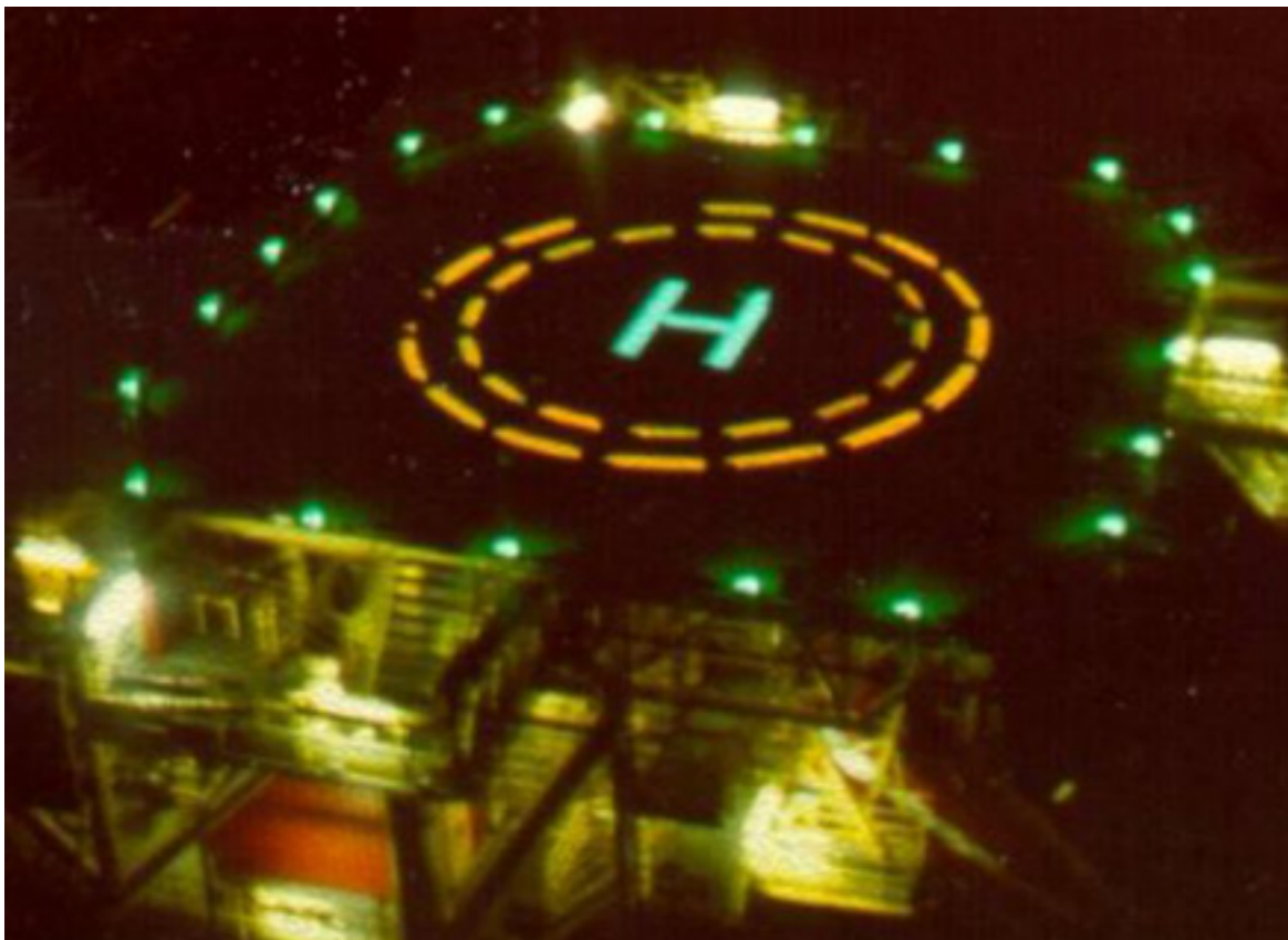
Figure 1 Photograph of preferred lighting configuration as determined by the trials performed at the NAM K14B platform [2]
