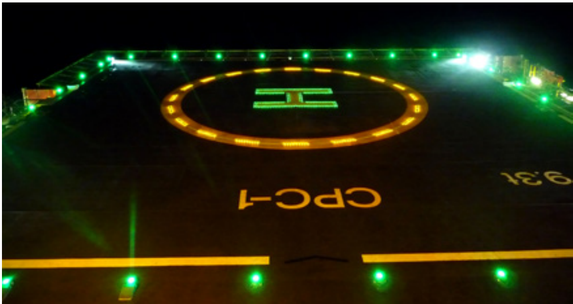
Figure 13 Touchdown/Positioning Marking circle segment on the CPC-1
