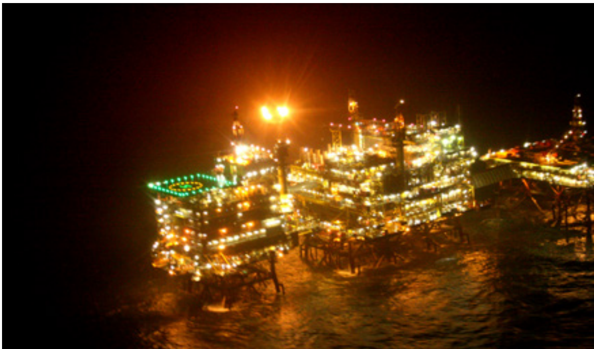
Figure 15 Aerial photograph of the AGI prototype lighting system on the CPC-1
