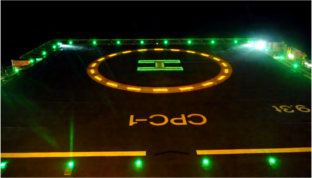
Figure 12 AGI prototype lighting system on the CPC-1
