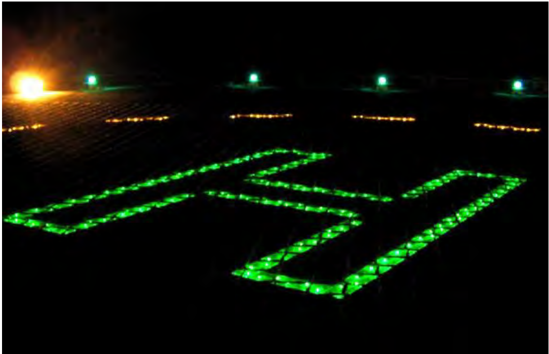
Figure 11 Helipoint Identification Marking ('H') on the Thames A
