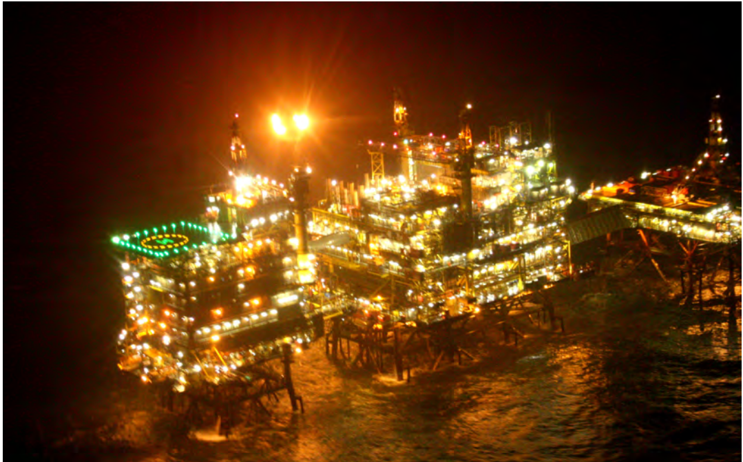
Figure 15 Aerial photograph of the AGI prototype lighting system on the CPC-1
