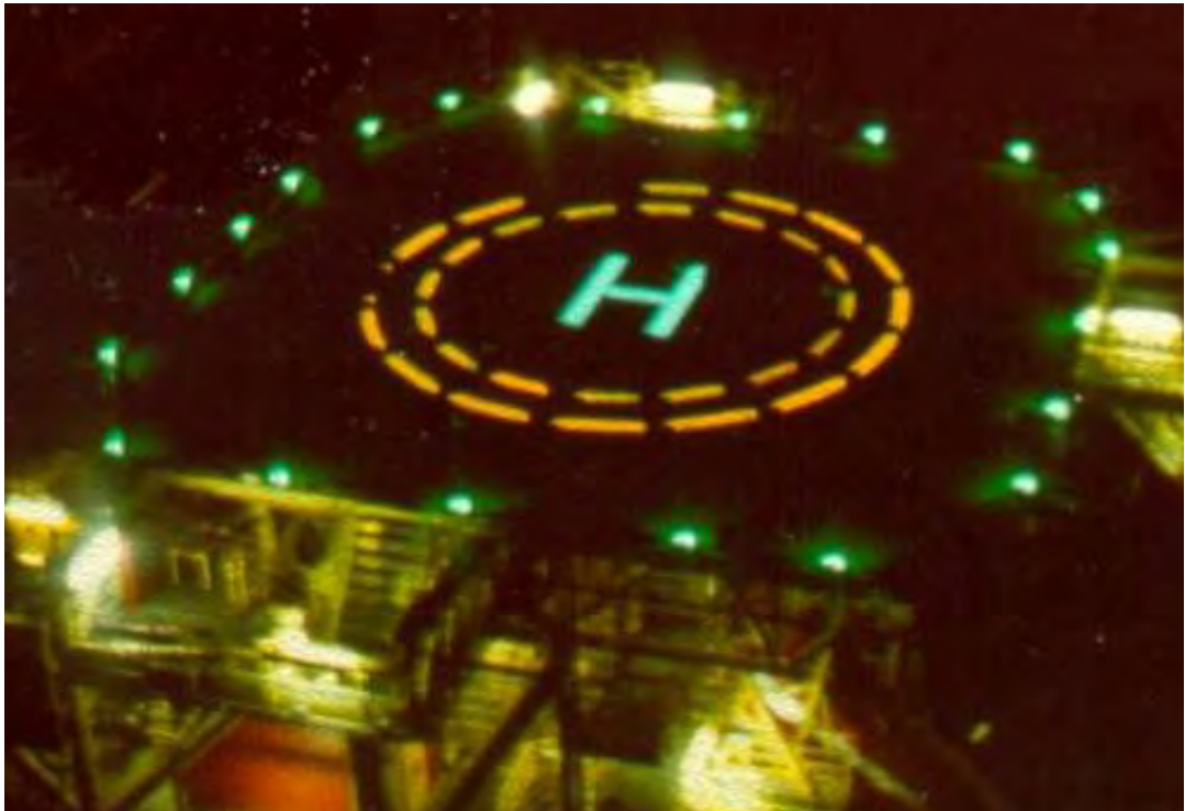
Figure 1 Photograph of preferred lighting configuration as determined by the trials performed at the NAM K14B platform [2]
