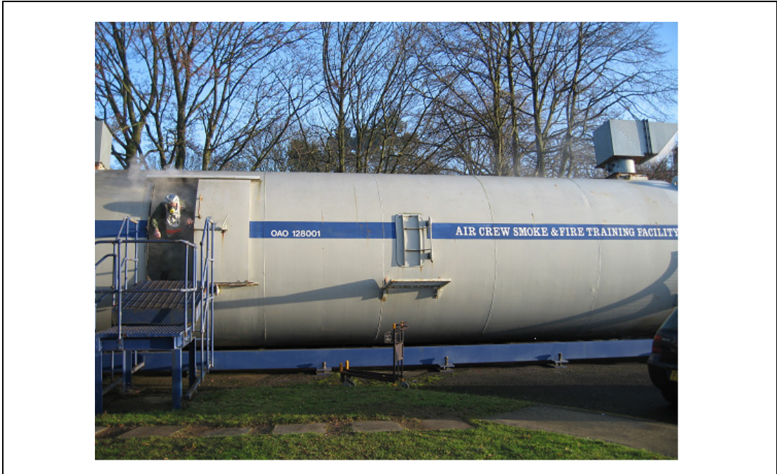
Figure 29 RAF Brize Norton Air Crew Smoke and Fire Training Facility
