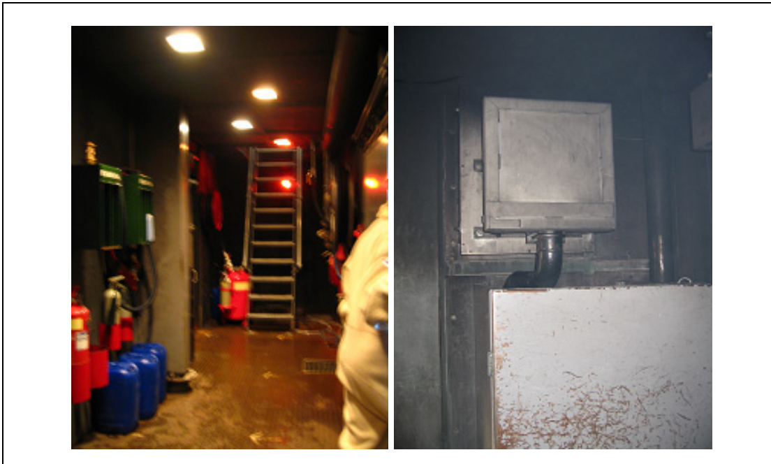
Figure 26 Passageway with Firefighting and Safety Equipment Stowage and Television Fire Rig on Middle Deck
