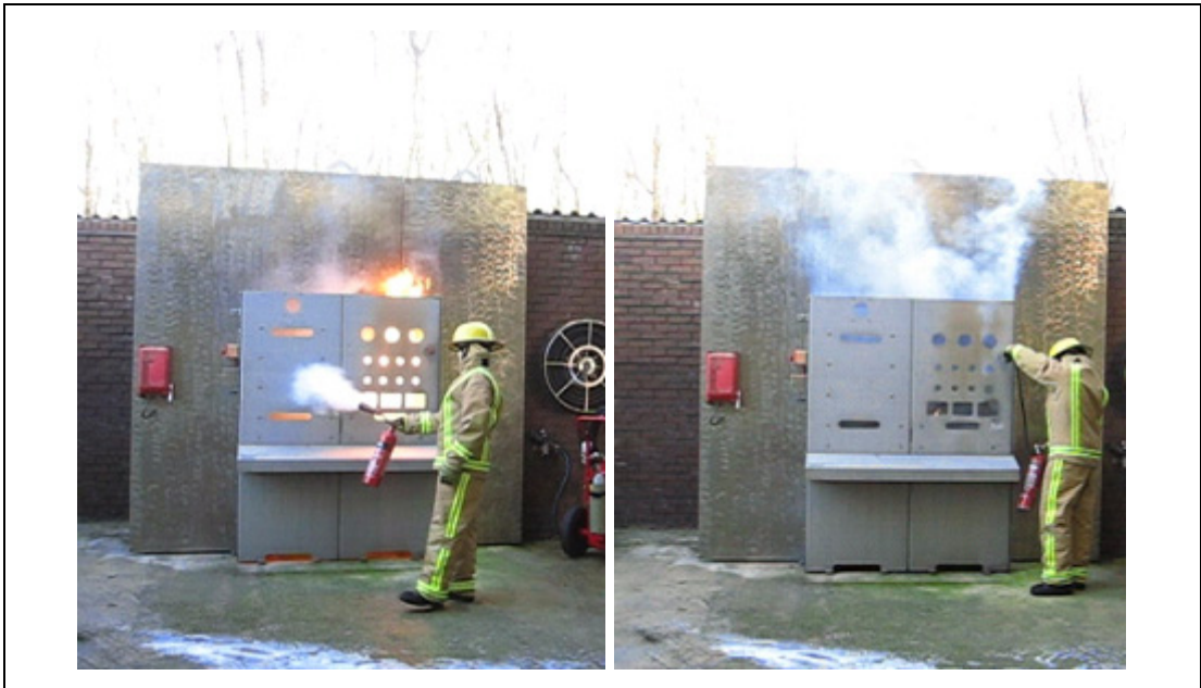
Figure 21 Demonstration of a Switchboard Fire Using a CO 2 Extinguisher (for Horn and Bayonet Fittings)
