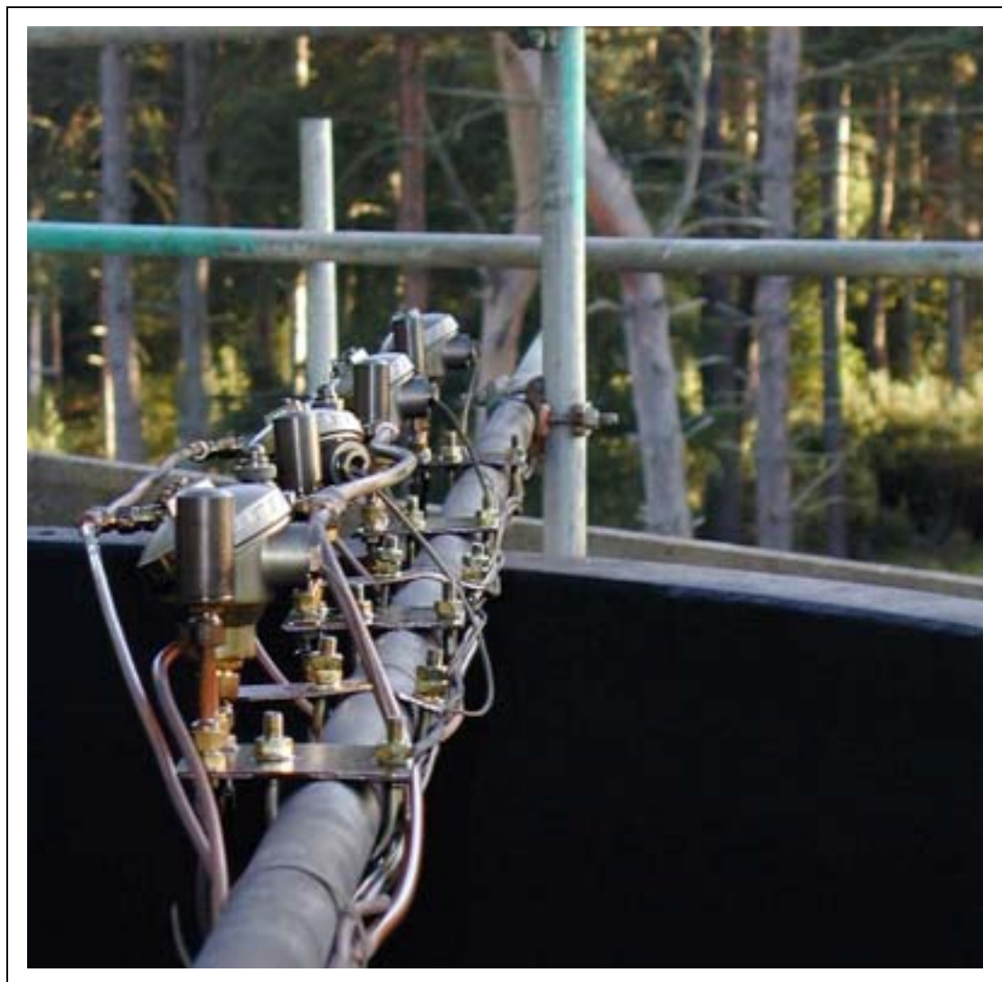
Figure 3 Spray boom with atomisers and instrumentation installed
