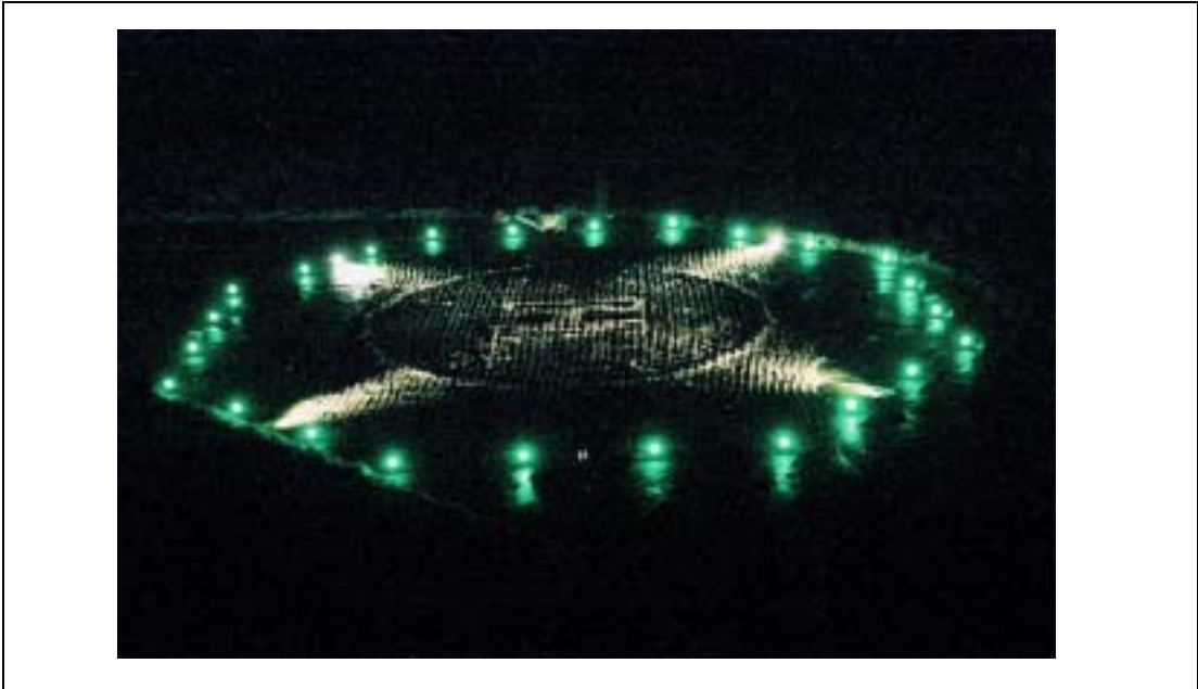
Figure 9 Deck-Level System Comprising Four Xenon Floodlights
