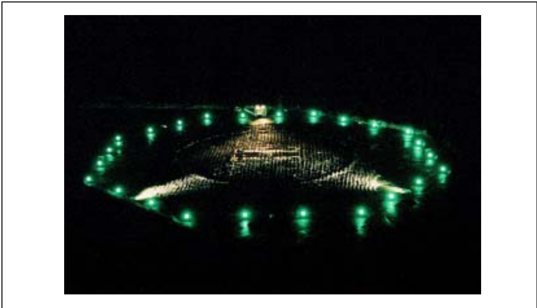
Figure 8 Combined High-Level and Deck-Level Configuration
