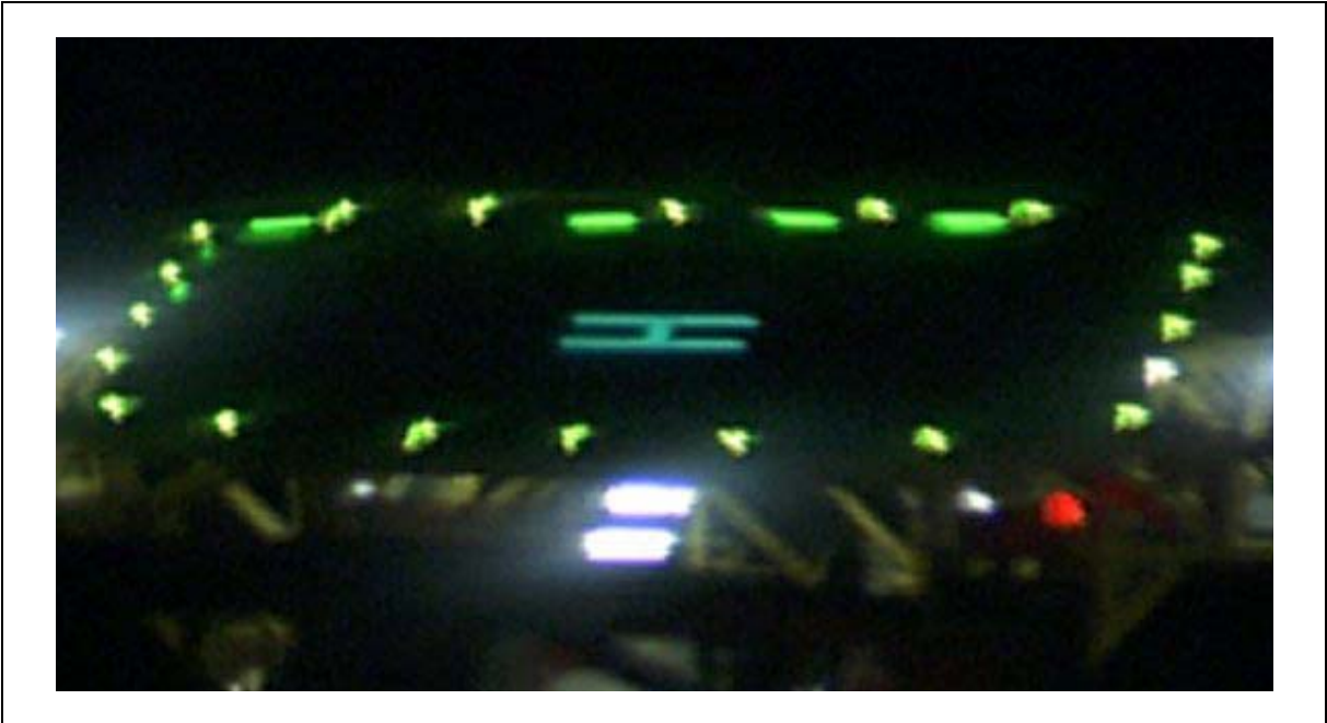
Figure 12 Green Light Emitting Diode Strips as Perimeter Markers
