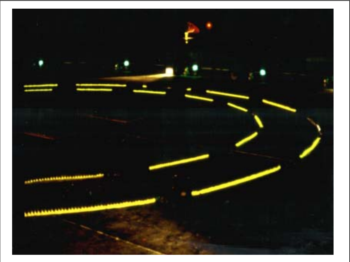
Figure 13 Yellow Light Emitting Diode Strips around the Touchdown Marking Circle
