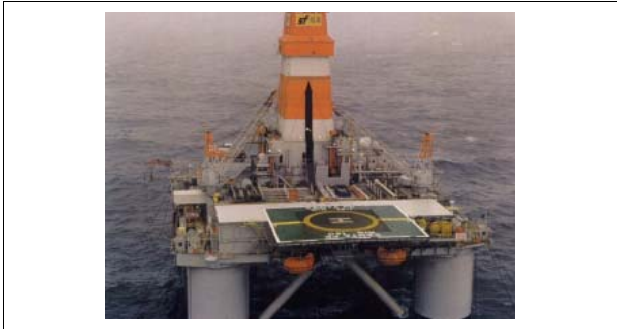
Figure 7.13 Santa Fe 140 Rig
