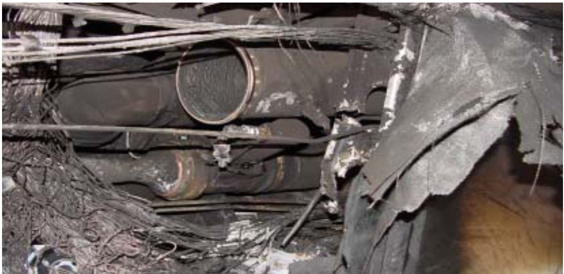
Figure 4 Fire in Cheek Area, Spread to Area Above Cargo Compartment
