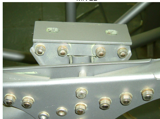
A port rear engine mount in a partly assembled aircraft showing the area of inspection on the outboard side of the brackets.
