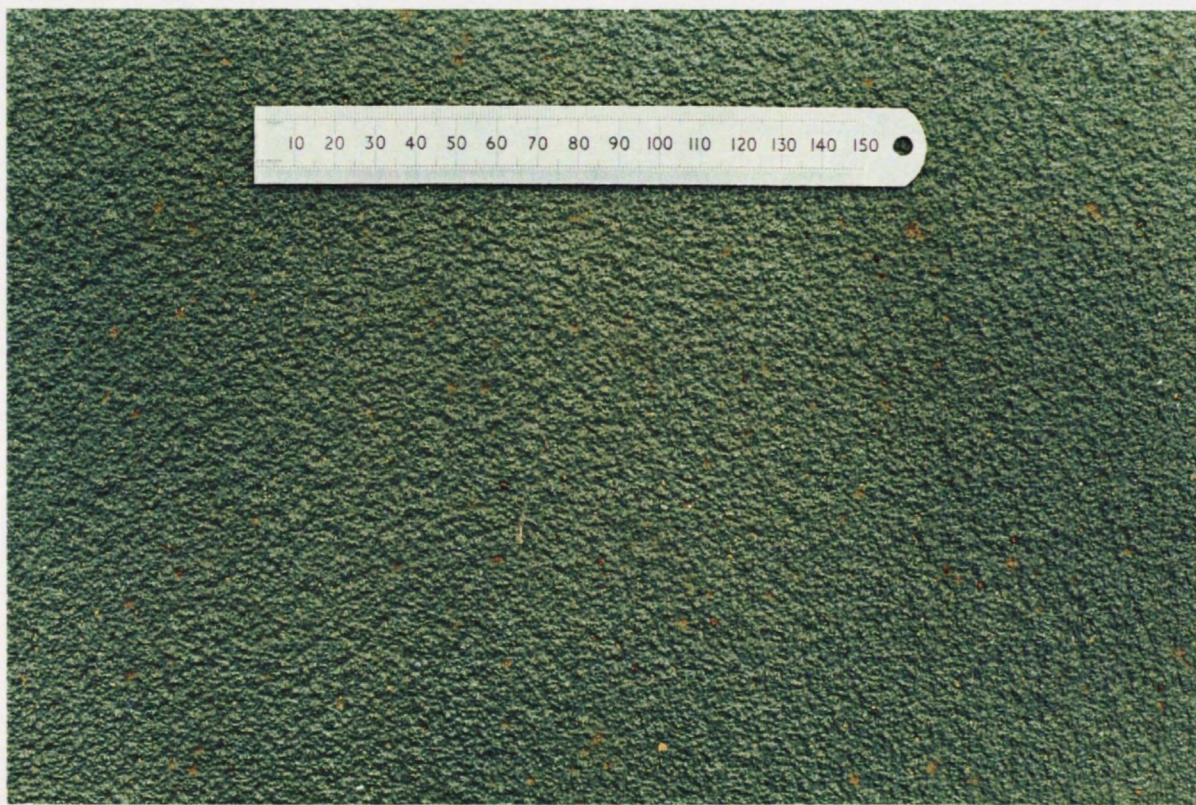
Figure 2 Sealcoat Green Deck Surface
